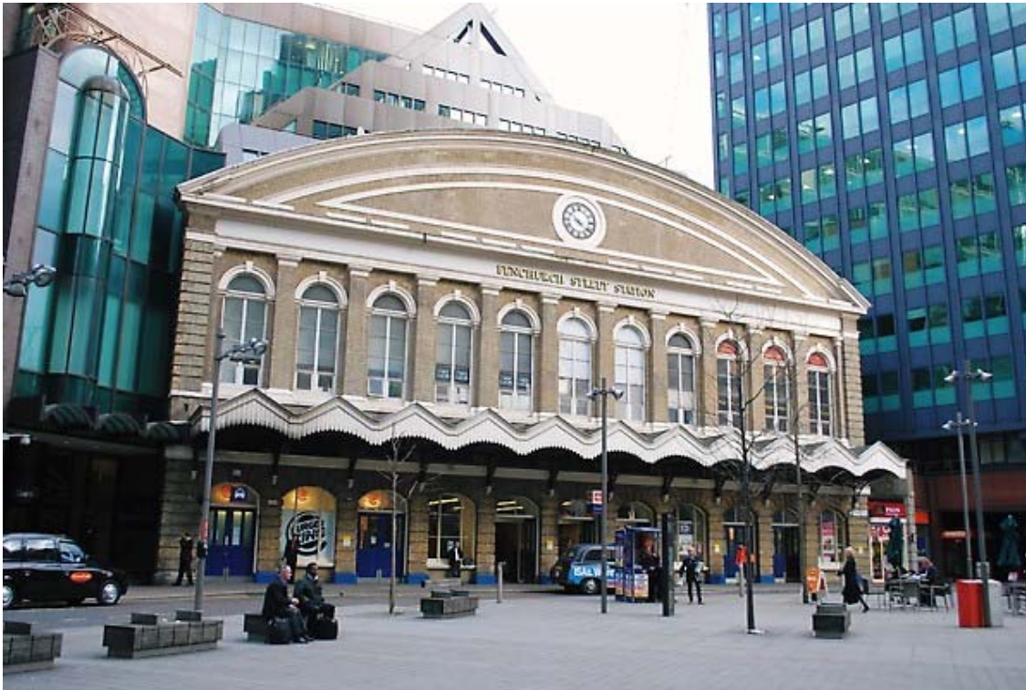
Fenchurch Street Station (EC3) has services running to destinations in east London and south Essex.
